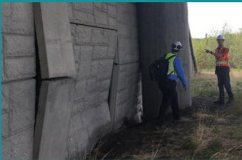
Proposed permanent repairs include reconstructing damaged roadway embankments plus replacing roadside hardware and repaving. Work on the damaged bridge will involve removing the panels, repairing damage to the retaining wall behind the panels, and re-hanging mended wall panels.
