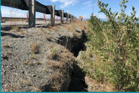
The November 30, 2018 earthquake caused roadway damage in multiple locations near the interchange of the Glenn and Parks Highways. Emergency repairs were performed immediately following the earthquake, with additional emergency repairs made in fall 2019. In August 2020, a Design Study Report was completed for proposed permanent repairs that, if approved, will be made during summer 2021.
